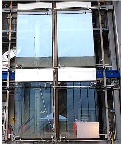
1. External view of the 4-unit specimen
